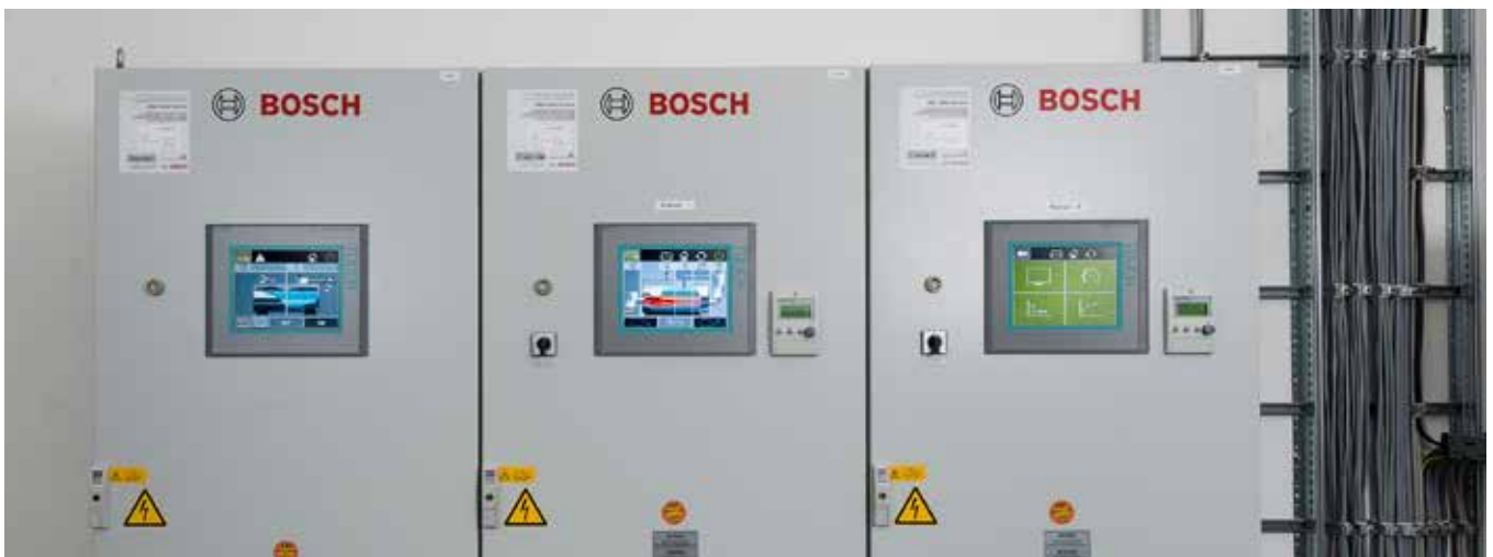
BCO boiler control with a preventive monitoring system ensures that there is a high level of transparency and simple boiler operation.
